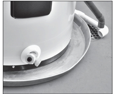
Figure 6 - A suitable drain pan piped to an adequate drain can help protect flooring from leaks and drips.
