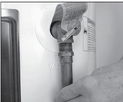
Removing the T&P Relief Valve discharge pipe.
